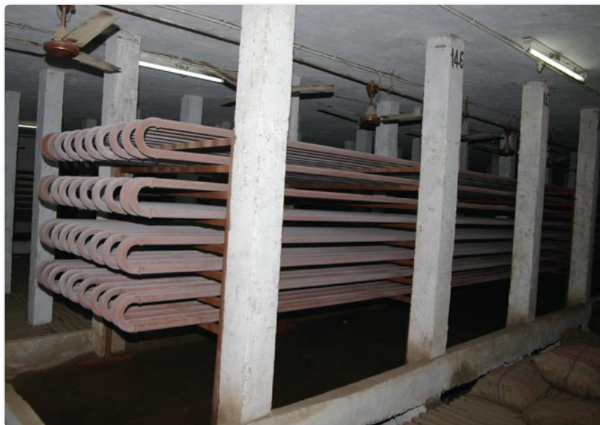
Bunker type potato refrigeration
